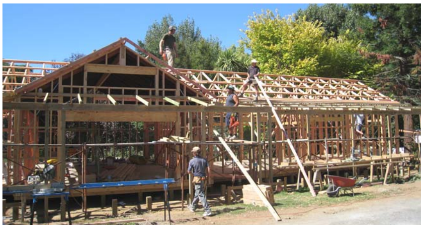
Above: Ian Cross painting the Taumarunui Anglican Church.
