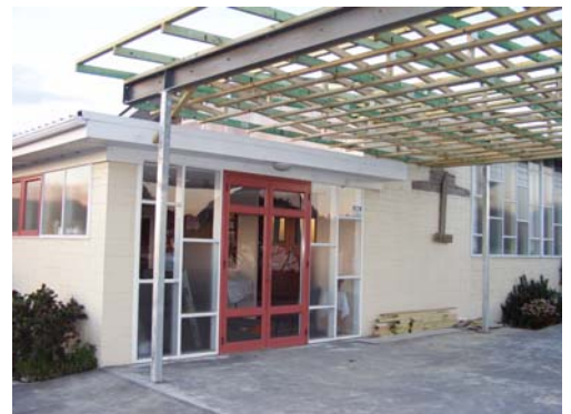
Huntly Baptist Church, new verandah
